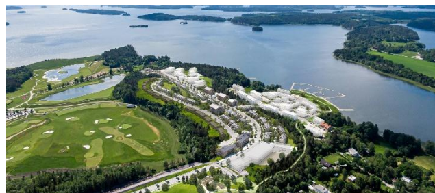
The Bro Mälarstrand project, stage 3, in Upplands Bro, comprises around 900 residencies from apartment buildings to detached and terraced houses with their own gardens.
