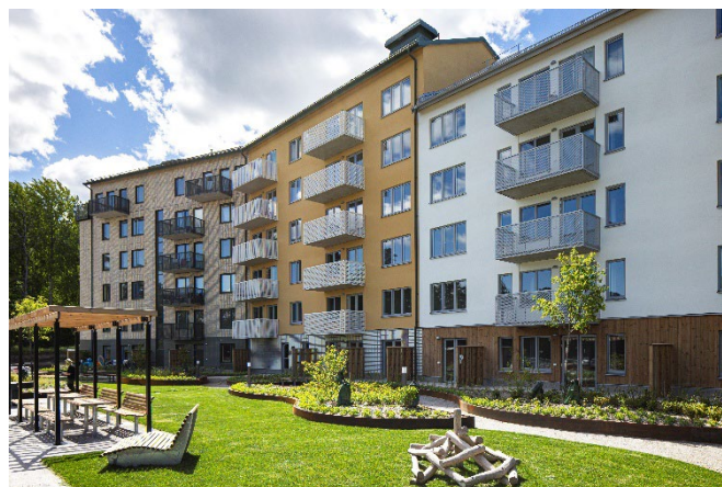
The Slagsta Strand project, stage 1, block 3.
