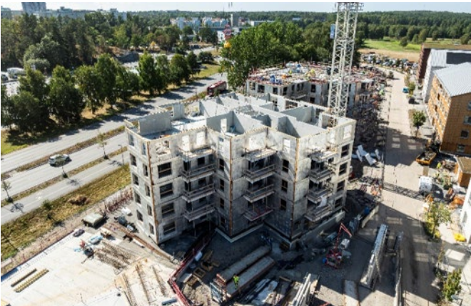
Bäverbäcken in Tyresö consists of 140 rental apartments and has been sold. Construction is well underway, and the project is expected to be completed during Q1 2028.
