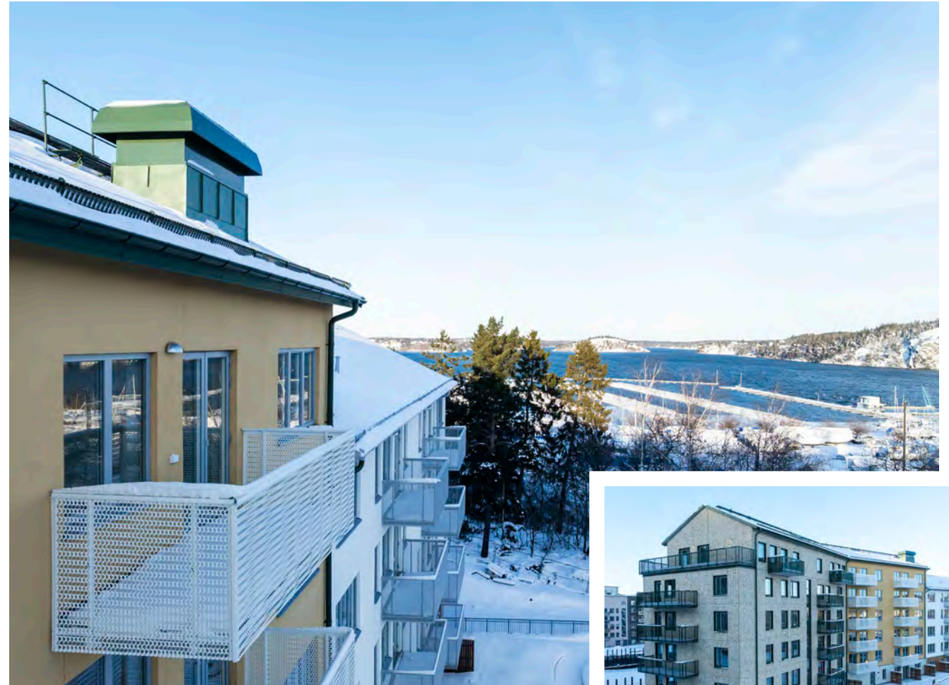
In a waterfront location next to Lake Mälaren in Slagsta Strand, Botkyrka, Magnolia Bostad has completed 77 space-efficient 1 - 4 bedroom apartments.
